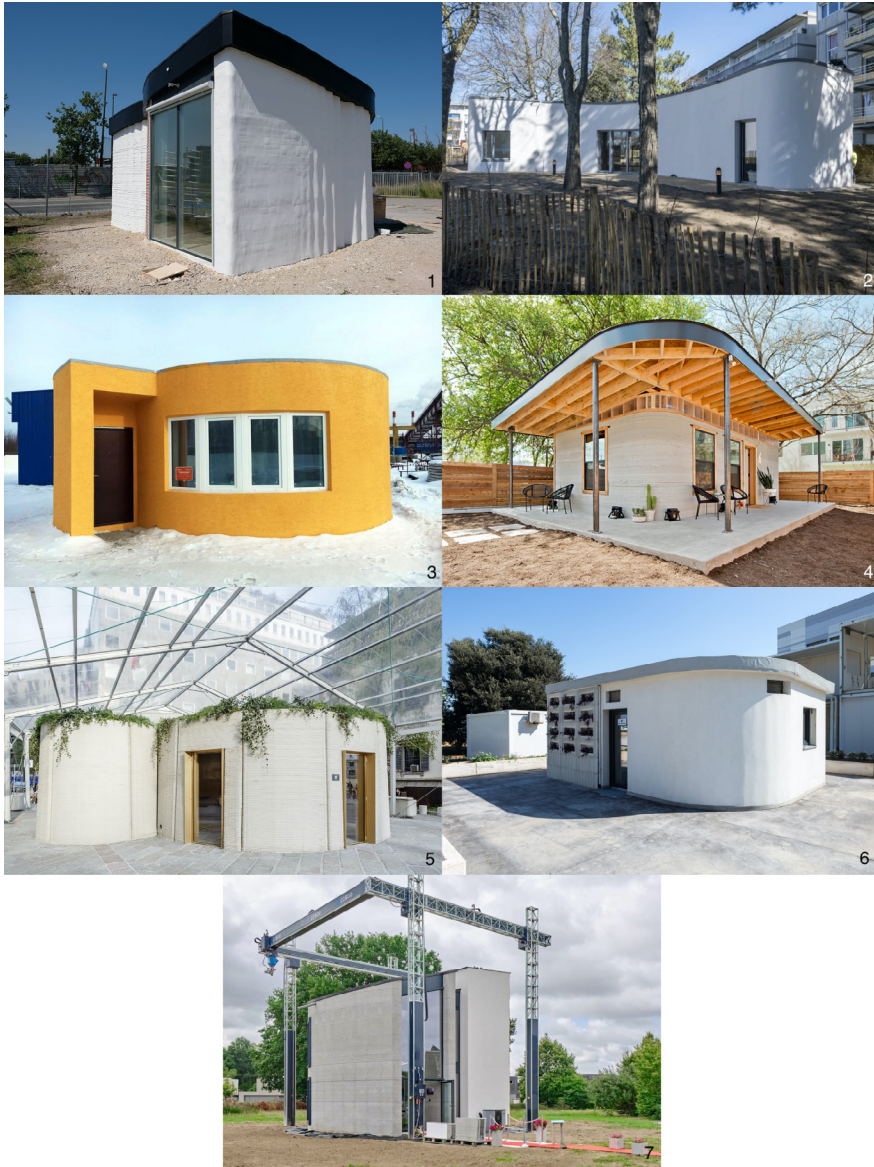
Imagen 2. Ejemplos de Viviendas Impresas (fuentes: https://cobod.com/the-bod/ ; https://theculturetrip.com/europe/france/articles/the-first-3d-printed-home-in-the-world-has-been-unveiled-in-france/ ; https://www.businessinsider.com/house-built-one-day-apis-cor-2017-3 ; https://www.archdaily.com/919667/could-3d-printing-be-the-future-of-social-housing ; https://bemore3d.com/language/en/3d-housing/ ; https://theurbandevolver.com/articles/portable-robot-prints-house-in-48-hours ; https://www.kampc.be/innovatie/projecten/3d-printen-in-de-bouw/presentaties-fotos , 2017-2020).
